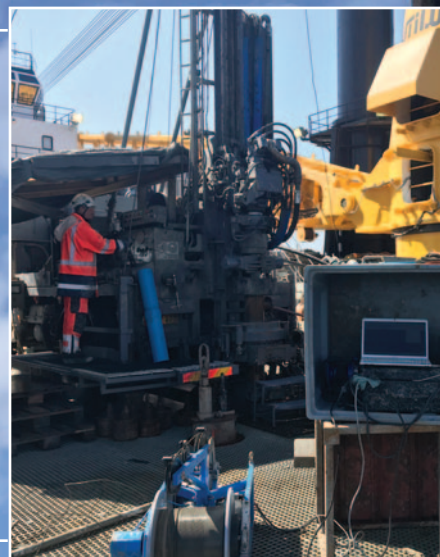
Robertson Geo's 2,000m marine winch secured to the drilling deck with the PS Logger® laid out to its left and ready to be deployed.
